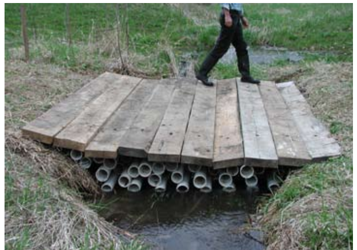
The Southwest Badger RC&D portable logging bridge was demonstrated at a Wisconsin Woodland Owners Field Day on May 05 near Fennimore.
